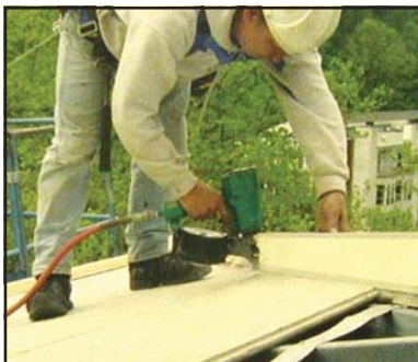
Nail to steel? ET&F's pneumatic nailing system makes fastening plywood to steel as fast as nailing to wood, resulting in substantial labor savings when compared to conventional screw fasteners.
