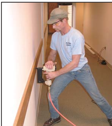
ET&F's Trimfast® pneumatic nailing system fastens interior and exterior molding and trim to light gauge steel as heavy as 14ga with finish nail-like fasteners for a quick, attractive installation.
