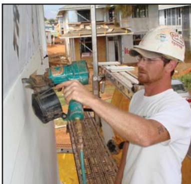
ET&F pins are code recognized for use attaching James Hardie® fiber cement siding to light gauge steel. See NER-405 for allowable design values.
