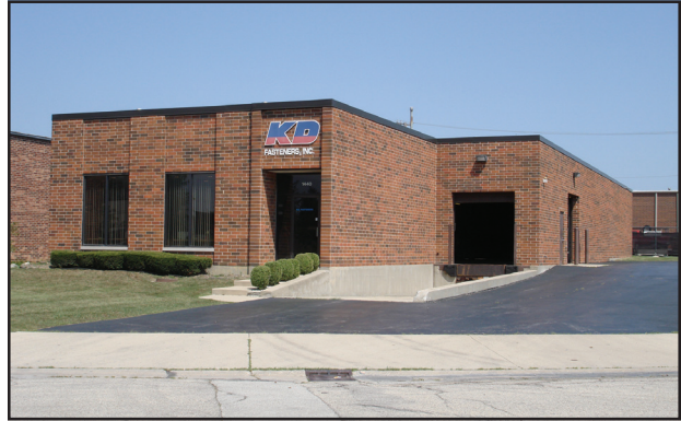
Kevin and Donna bought the building in 1990. It is located at 1440 Jeffery Drive in Addison, Illinois
